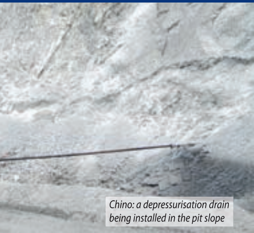
Prism data was used to manage the slope and demonstrated the benefit of the slope drains
